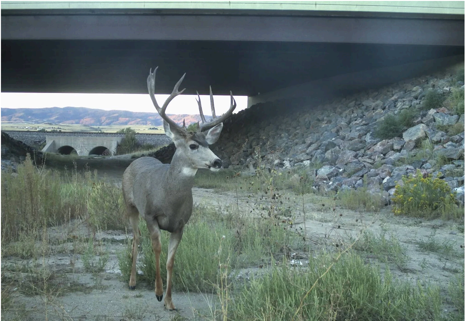
Deer using wildlife underpass beneath US 85 near Sedalia, CO. (Another highway underpass can be seen in the background.) ©CO Dept of Transportation
